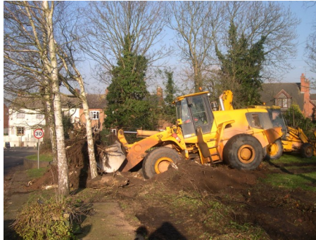
Work starts on the green 2006
