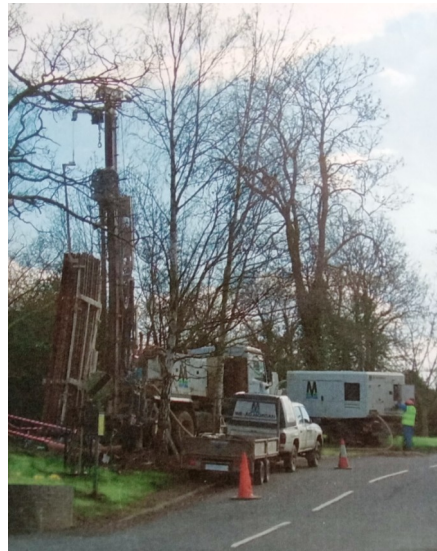
Well head drilling 2007
